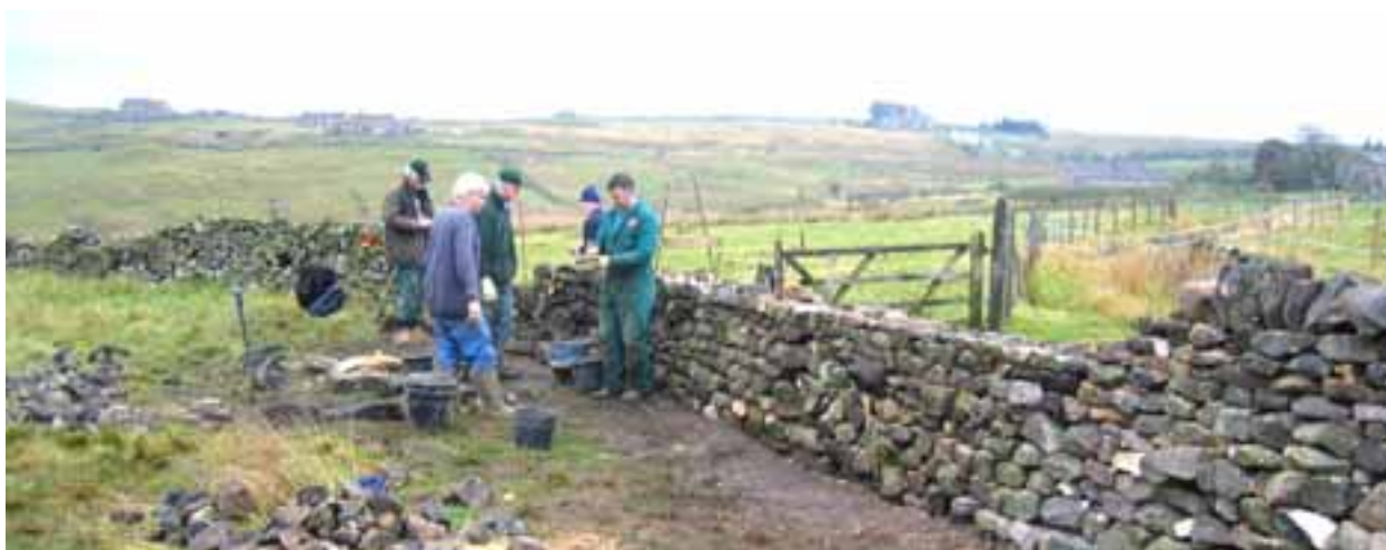
Drystone wall building at Greenhow.
