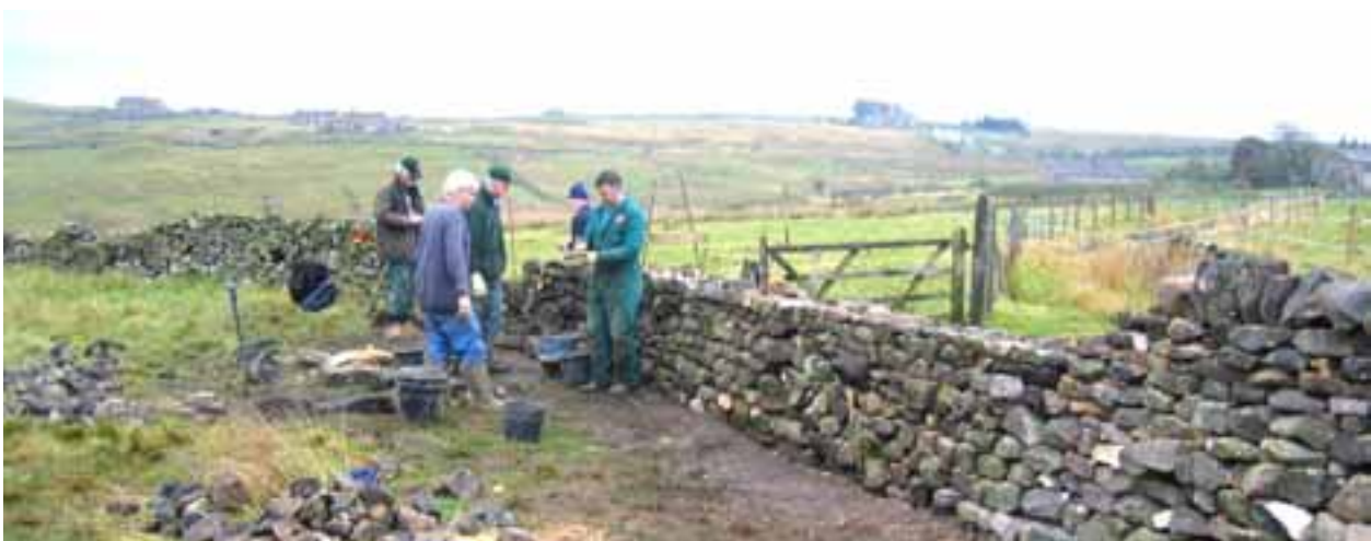
Drystone wall building at Greenhow.
