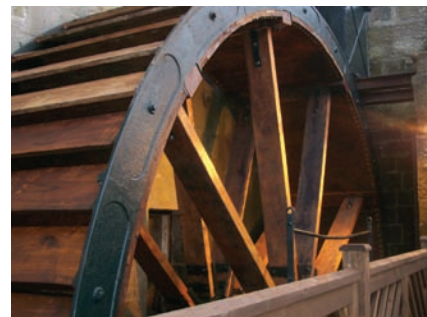
The newly restored water wheel.
