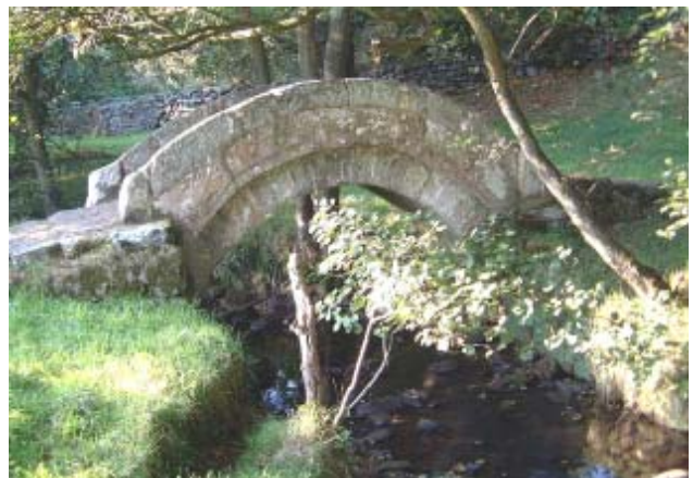
Dacre Packhorse bridge
